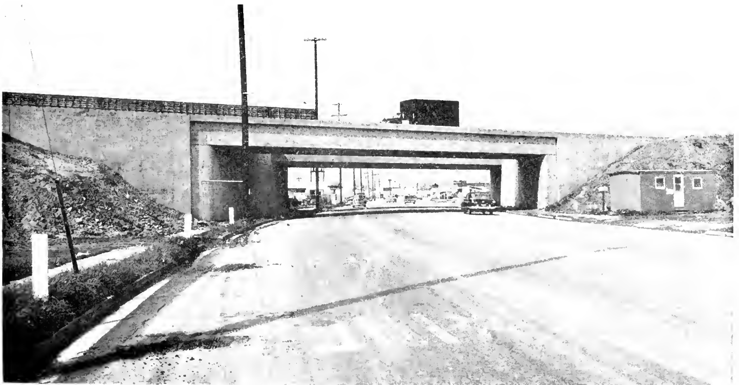
East Market Street separation structure under construction, looking westerly, now completed.
